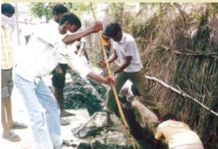
Cleaning of side canals at Peddavaram
